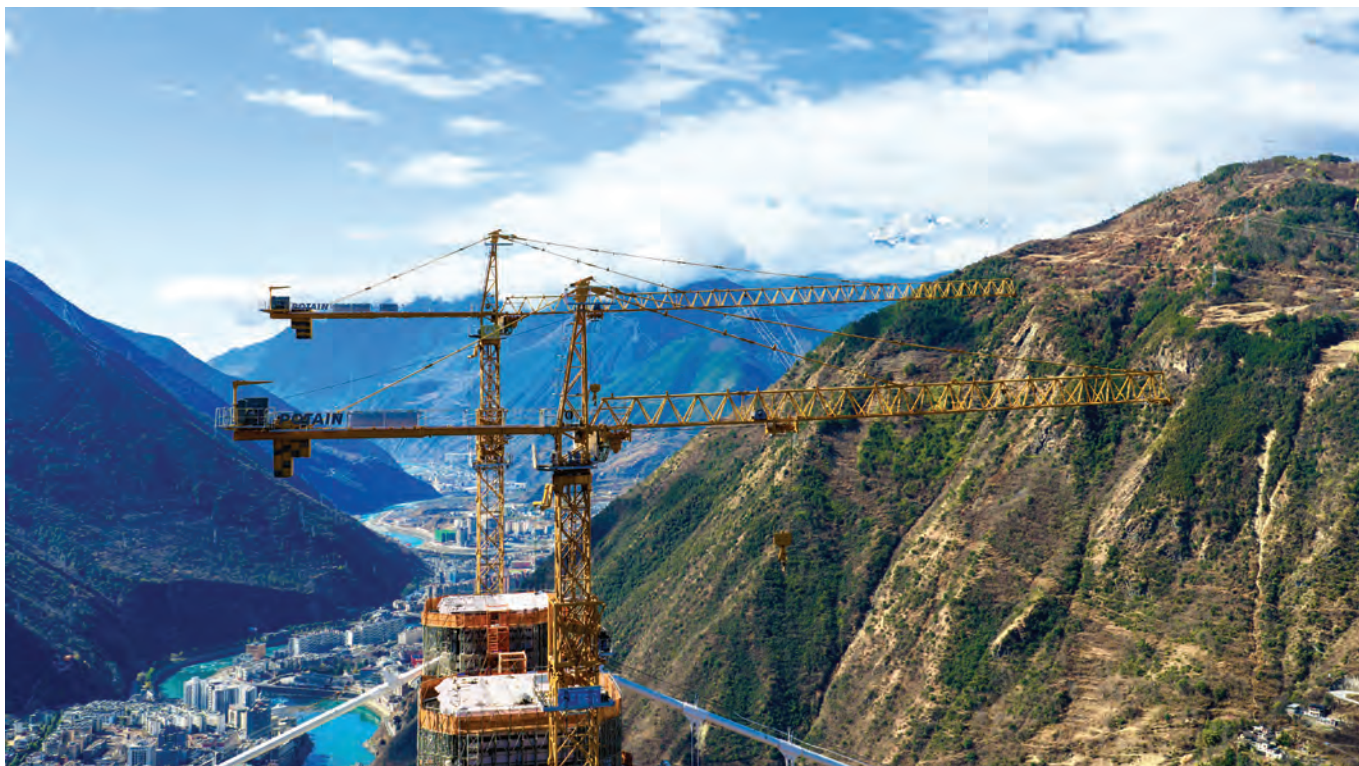
ABOVE AND LEFT: Three Potain MC 480 tower cranes helped construct the bridge's pylons, working under extreme conditions that included a deep V-shaped canyon and strong winds.
