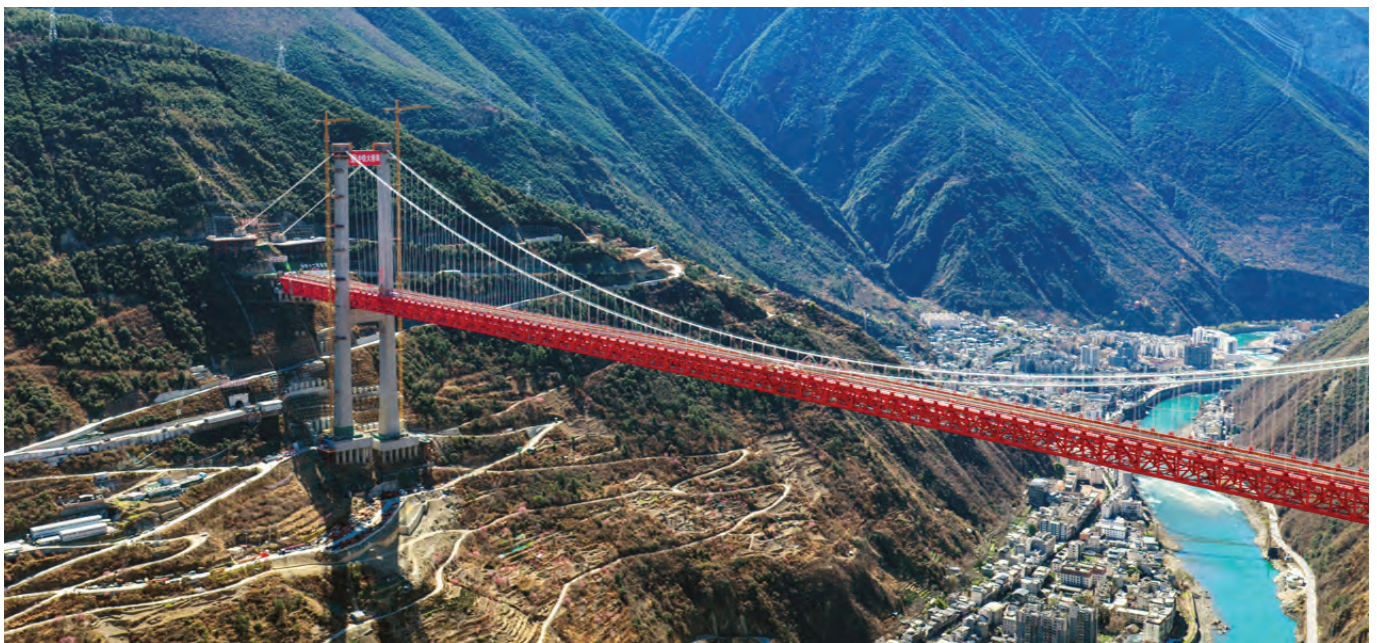
TOP AND ABOVE: The new 1,060 m bridge, part of the Sichuan–Tibet Railway, is being built to improve connectivity across the local mountainous terrain.
