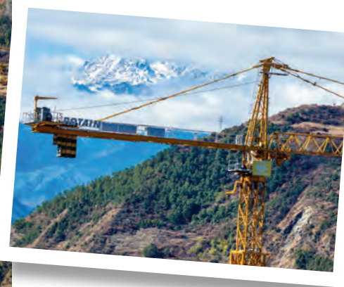
BELOW: The cranes were configured with jib lengths ranging from 40 m to 60 m and operated at their full 25 t lifting capacity.
