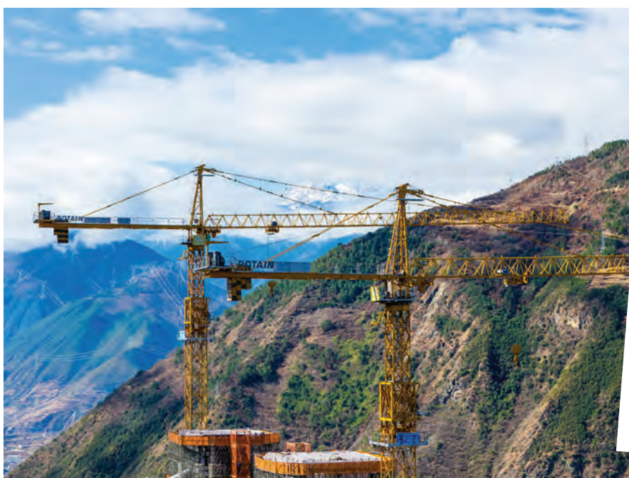
ABOVE AND LEFT: Three Potain MC 480 tower cranes helped construct the bridge's pylons, working under extreme conditions that included a deep V-shaped canyon and strong winds.
